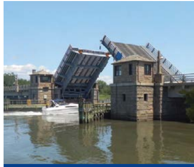
Bayville Bridge Rehabilitation (Bayville, NY) GOLD AWARD
