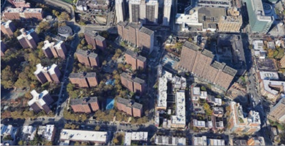
NYCHA Eastchester and Jackson Houses Design Build - Geothermal DHW and Heating Upgrade | Platinum Award
