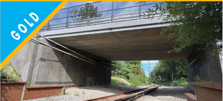
Webster Avenue Bridge Replacement
