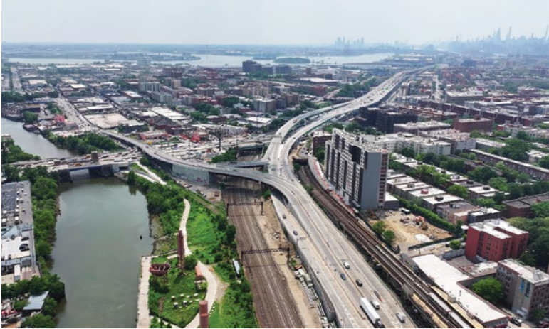
Transforming the Bronx: The Hunts Point Interstate Access Improvement Project (Bronx, NY) DIAMOND AWARD
