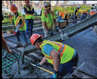
The Backbone of Brooklyn, Innovative BQE Repairs Project (NYCDOT)
