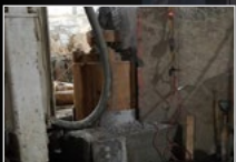
Drilling of 36-inch Diameter Caissons within Building
