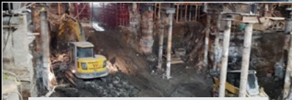
Foundation Support and Excavation below Landmark Theatre
