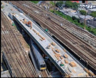
LIRR Hall Interlocking Expansion Project (MTA C&D)
