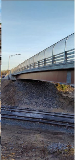
Kings Road Bridge Replacement | Silver Award
