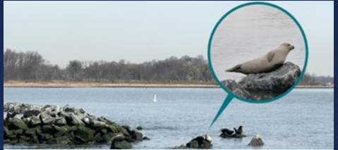
Harbor seals spotted on partially constructed breakwater.
