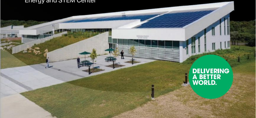
Suffolk County Community College, Design Services for Renewable Energy and STEM Center
