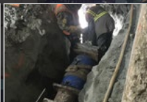
Lateral Testing for Caissons up to 1,160 kips
