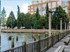
Construction Management Battery Park City Authority South Cove Quay Storm Damage Repair
