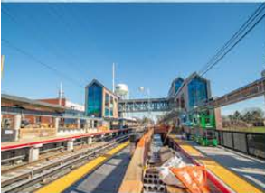
Design Build MTA Long Island Rail Road Third Track Expansion
