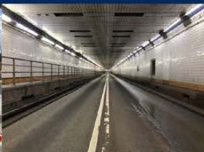
Inspections Port Authority of NY and NJ Holland Tunnel Biennial Inspection
