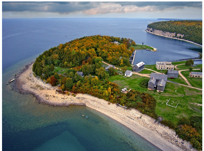
Figure 9: Fayette townsite, Snail Shell Harbor, and the Middle Bluff cliffs. Photo provided by Fayette Historic State Park.
