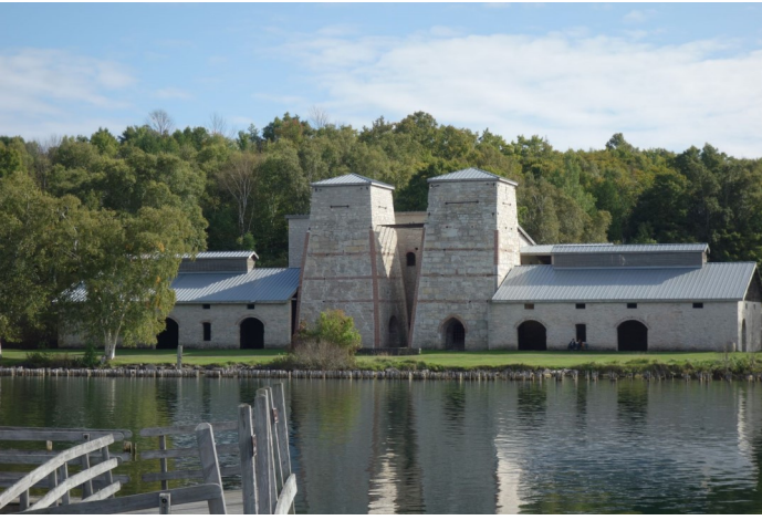
Figure 10: Remains of the Fayette blast furnaces. Photo by Dave Adler.
