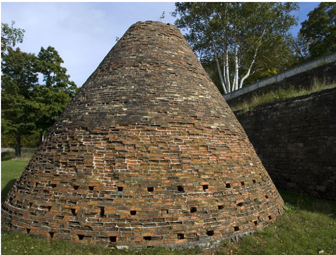
Figure 11: Kiln used for converting wood to charcoal. Photo provided by Fayette Historic State Park.
