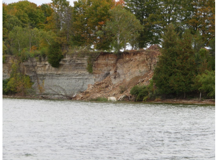
Figure 18: Bedrock Cliff Collapse where the Bill's Creek Shale has undercut the Overhanging Stonington Limestone North of Stop 3. Photo by Dave Adler.
