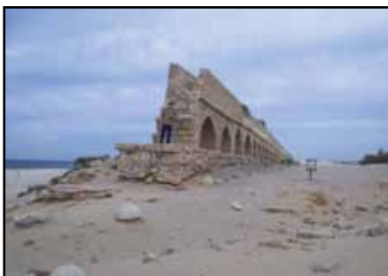
Figure 8. The Roman aqueduct at Caesarea constructed using the Kurkar Sandstone. Author is shown for scale.
