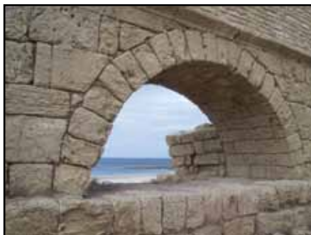
Figure 9. Portal in aqueduct above showing close-up of Kurkar Sandstone.
