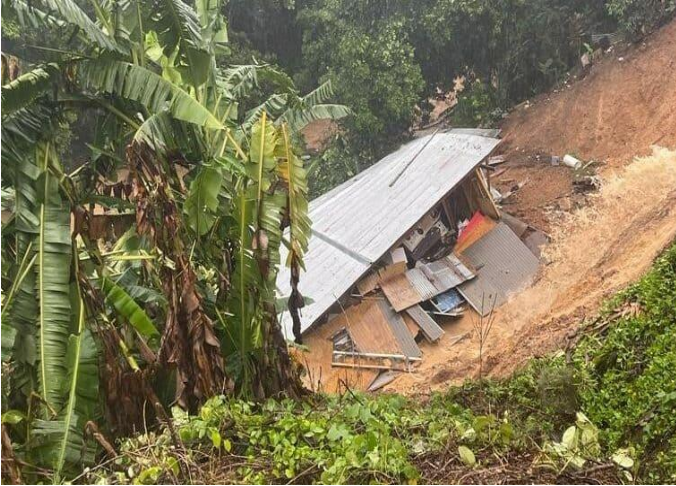
Landslide damage. Barranquitas, Puerto Rico
