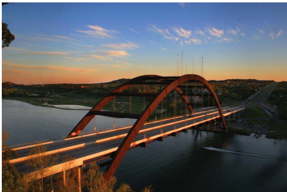
Loop 360 Bridge at Sunset
