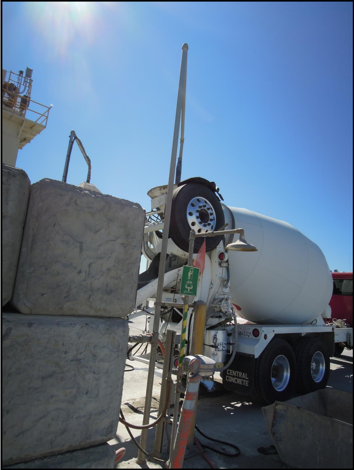
Ready Mix Truck Receiving Reclaimed Water for Washout
