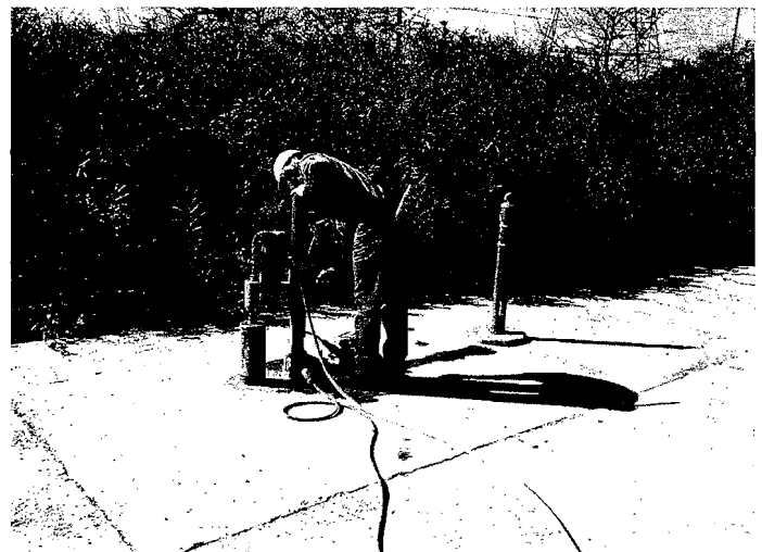
Figure 4. Coring concrete cylinders.
