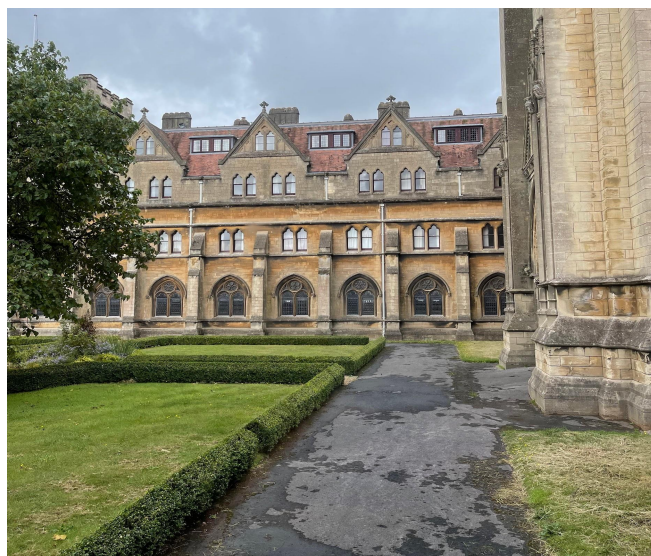
Figure 3: A view of part of the monastery built by Dunn and Hansom begun in 1873. Courtesy of the author.
