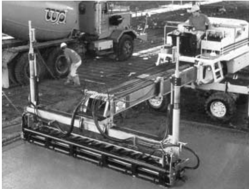
Figure 4.2 A laserscreed machine at work
