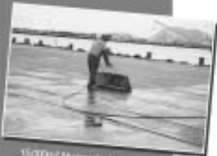
15000m 2 Airport tarmac Aquoron 7000 chloride protection.
