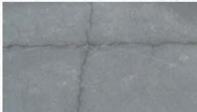
Figure 3: Settlement Cracking
