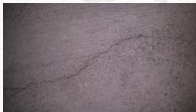
Figure 1: Plastic shrinkage cracking
