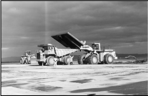
Front End Loaders Lifting a Slab
