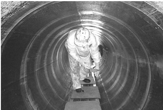
Figure 4 – Internal view of repaired pipe.
