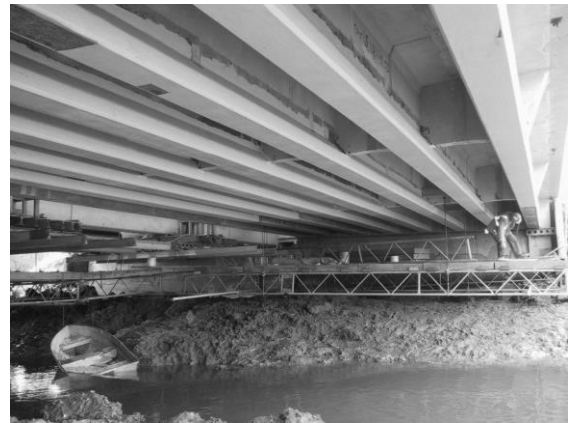
Figure 3 – Esmonde Rd bridge girders after wrapping with FRP
