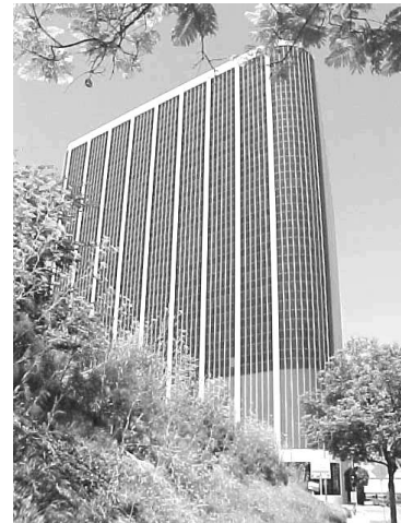
Figure 1 – Building at 333 South Beaudry Ave, Los Angeles
