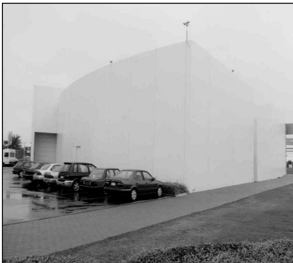
Figure 2: View of Concrete Panels Relocated to Form Extension
