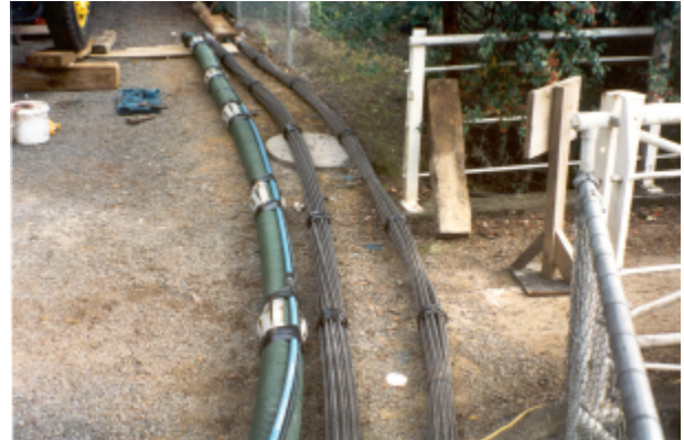
Figure 8: Strand anchor arrangement
