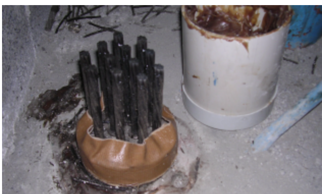
Figure 13: Strand anchor head prepared for protection
