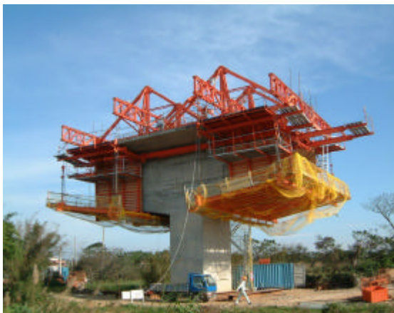
Photo: 1. VSL MODULAR FORM TRAVELER - C215 High Speed Rail - Taiwan
