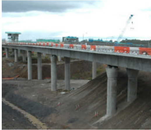
Figure 3 – Elliptical Column Heads
