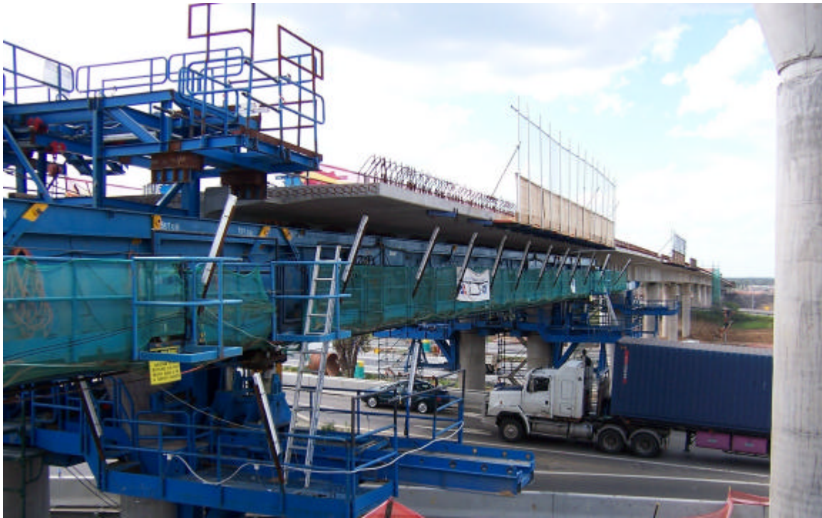
Figure 8 – Gantry for Span by Span Bridges
