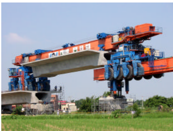
Photo 4. High Speed Rail Project, Taiwan
