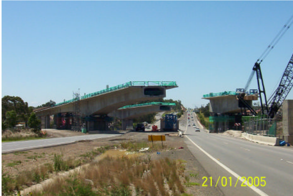
Figure 9 – Balanced Cantilever (Old Windsor Road)
