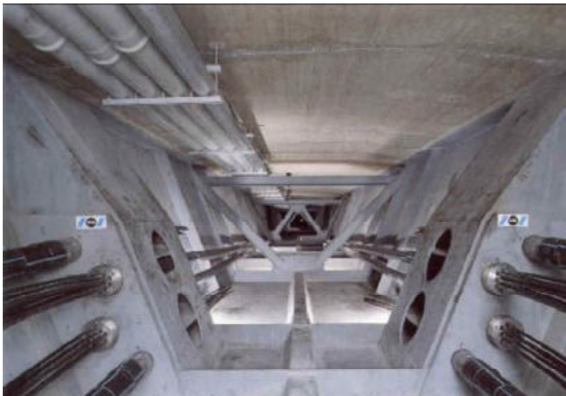
Above View : External Post-Tensioning Inside Bridge Segment
