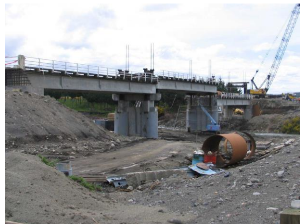
Bridge deck at 3 Different levels
