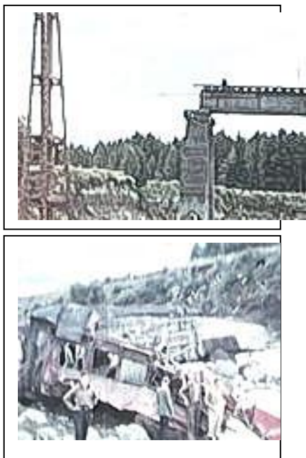
Photos following 1953 Railway disaster
