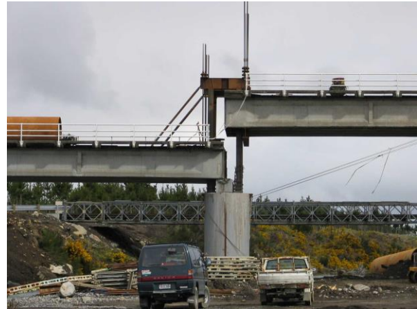
Central span in lifted position
