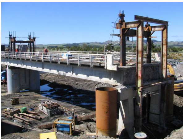
Abutment lifting arrangement
