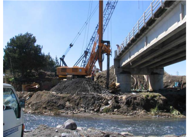
Clearing out casing
