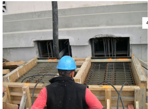
Fig 11. SCC Concreting of the Drop-Down Beams
