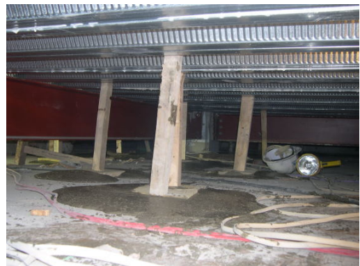
Fig 7. Quality Control Inspection Holes in Action
