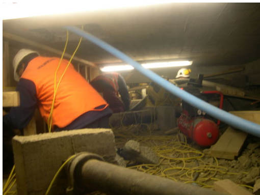
Fig 6. Construction of the Beam Formwork
