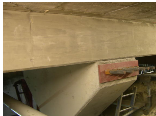
Fig 13. Completed Beam and Column Cap
