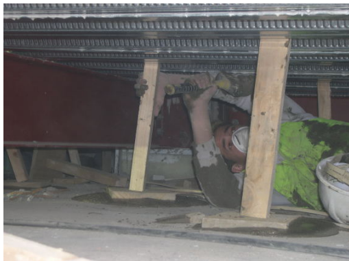
Fig 12. Blocking the Inspection Holes
