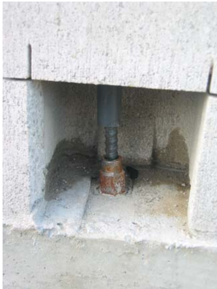
(c) Tendon coupler at floor height prior to grouting
