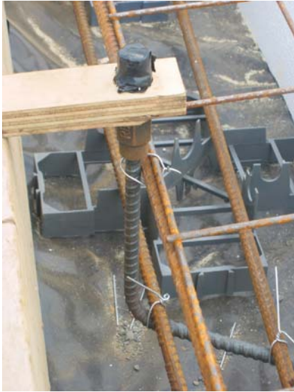
(a) Tendon anchorage in exterior beam
