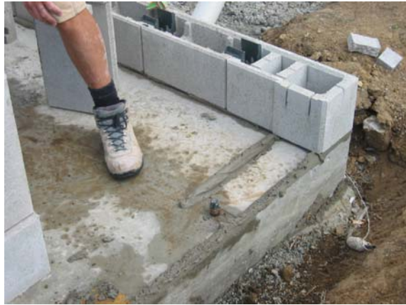
(b) Laying the first course of blocks
