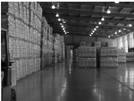
Figure 4 – Finished storehouse in use
