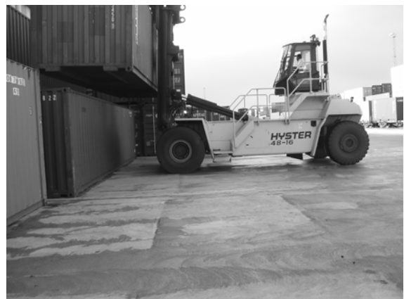
Figure 6 Container lifting equipment with 84 tonne axle loads operate on the post-tensioned concrete pavement
