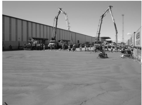
Figure 5 The external pavement during construction.
