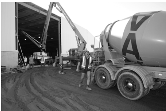
Figure 15 Concrete is discharged into a pump at a doorway
