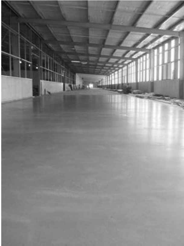
Figure 7 The 460 m railway unloading tunnel.
