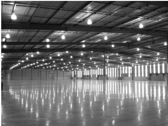
Figure 1 Finished internal storehouse floor
