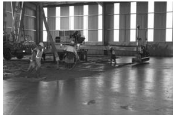
Figure 2 Somero Laser Screed in use for internal storehouse construction
