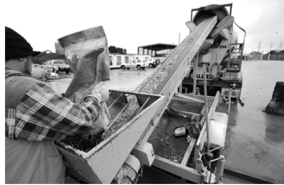
Figure 9 Xorex steel fibre loaded into a ready mixed concrete truck
