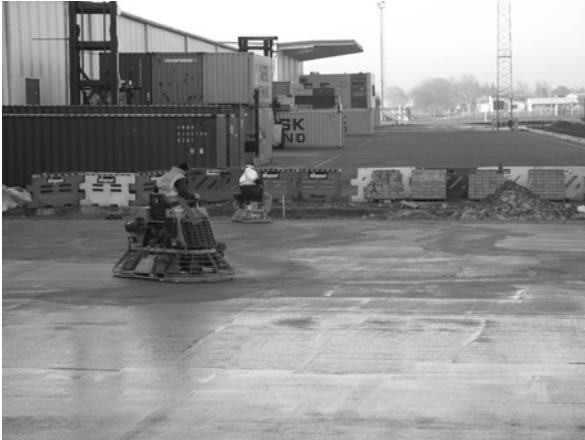
Figure 17 Large container stand pour during finishing.
