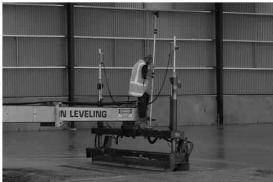
Figure 5 Technology such as Somero Laser guided screeds, can be used to increase control of surface regularity
