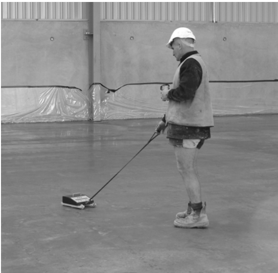
Figure 10 A “F meter” device rolls along the floor taking semi-continuous measurements of elevation.
