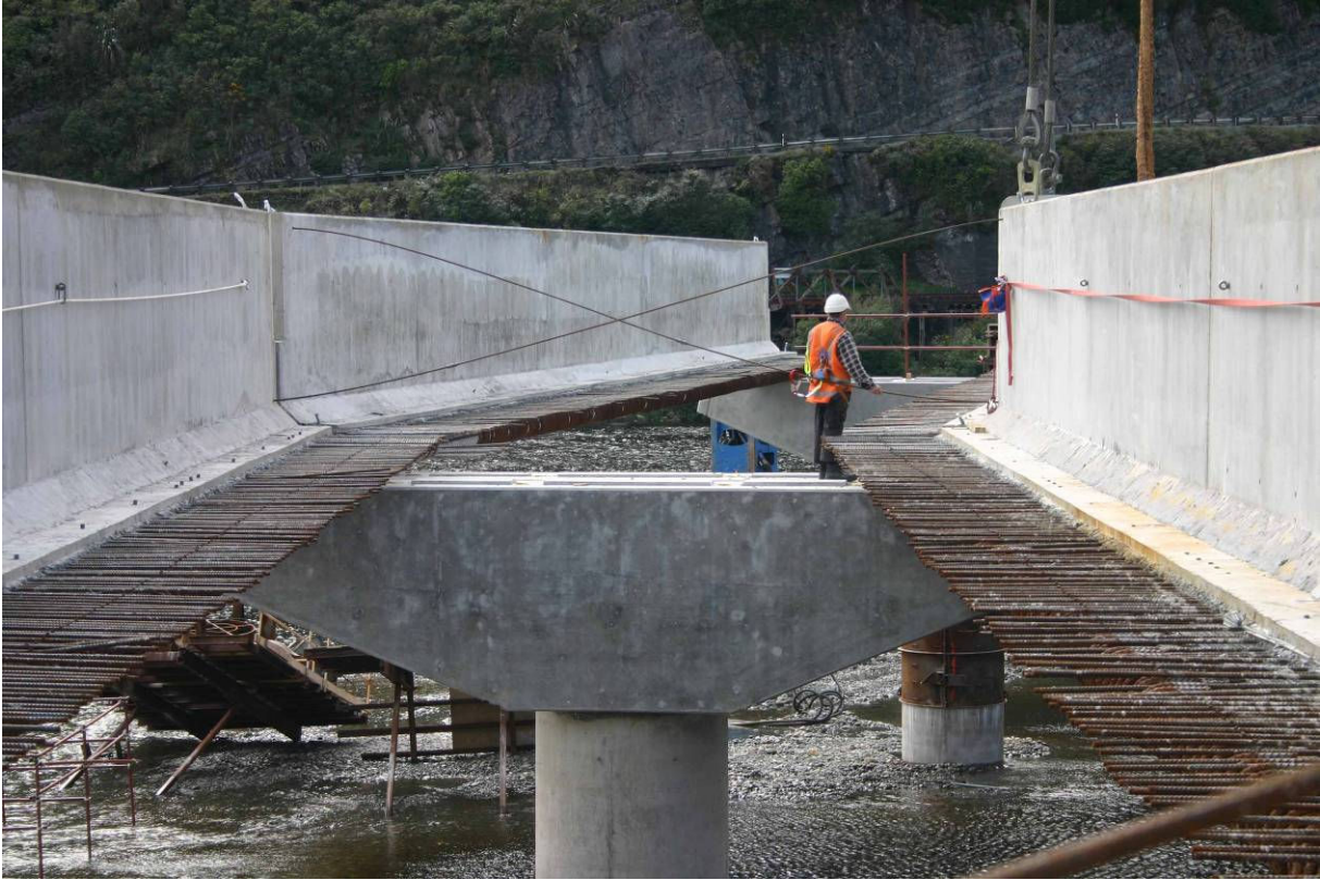
Figure 4 Precast L-beams in place on piers
