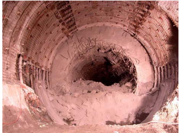
Pic. 11 Re-profiling using 'flexible' Rock Support
