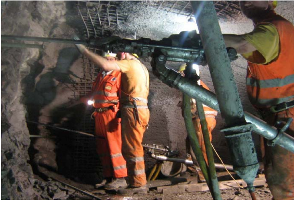
Pic. 4 Hand Mining over Top Shield
