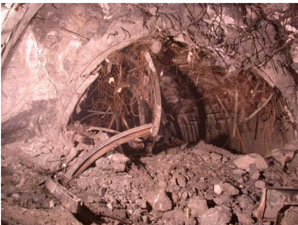
Pic. 10 Destruction of 'rigid' Rock Support
