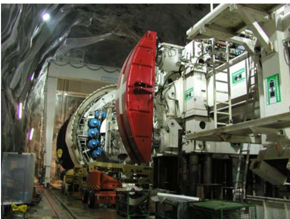
Pic. 2 TBM Assembly inside Cavern
