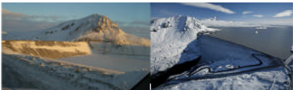
Figure 3: January 2007 and January 2008 Concrete faced rock filling dam after start of filling with water and at full water level
