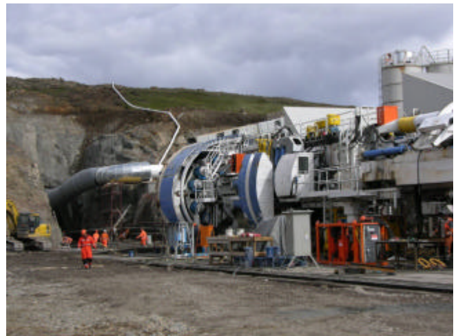
Figure 1: Assembled TBM2 ready to be moved to the start for drilling
