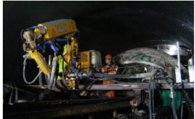
Figure 5: Shotcrete manipulator on the back up of the TBM
