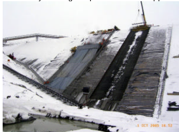
Figure 5: Concrete face slab: concreting under extreme winter conditions
