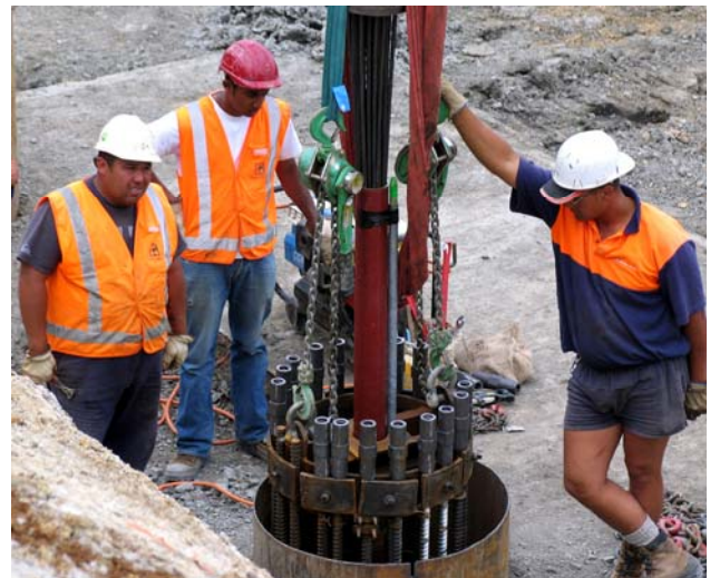
Figure 2. Placing stressing tendons in the western abutment piles
