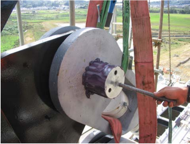
Figure 13. Inserting the clevis pin.
