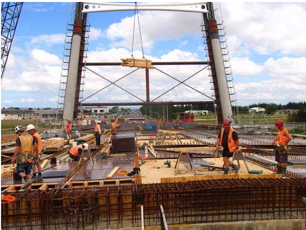
Figure 8. Construction of the insitu concrete deck
