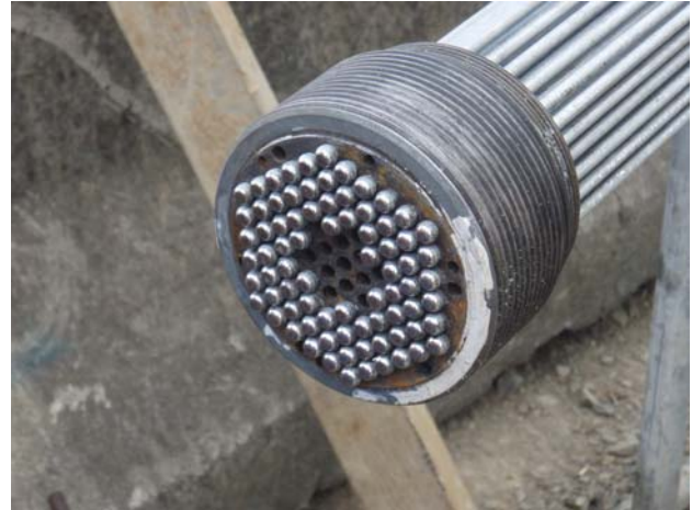
Figure 11. Wires terminated with button heads at an end anchorage
