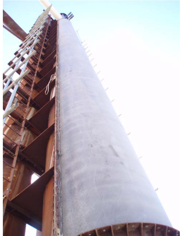
Figure 6. Stripped top section of the pylons
