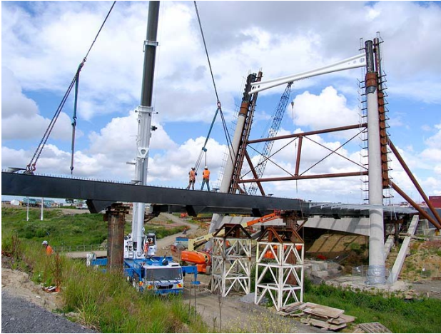
Figure 7. Erection of eastern half of the box girder
