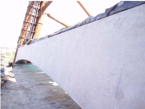
Figure 5. Curved concrete crossbeam which supports the bridge deck at the pylons
