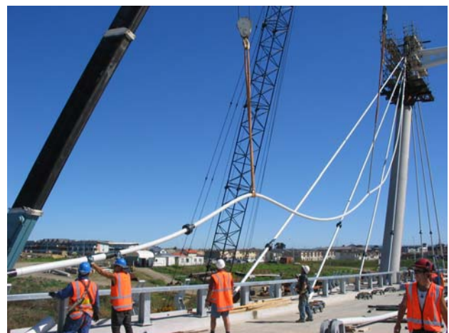
Figure 12. A stay being installed using a three point lift system
