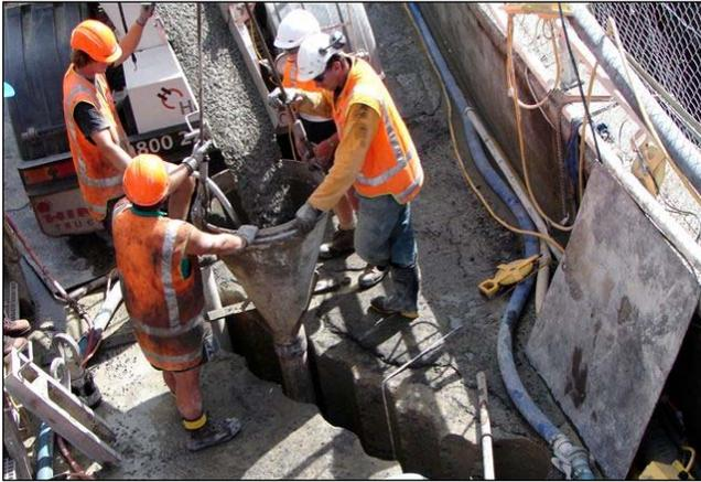
**Figure 2: Discharging Concrete into Tremmie Funnel**
