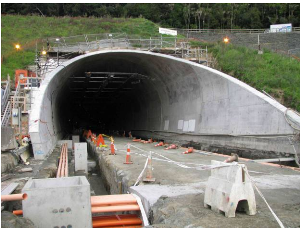
Figure 11: Johnstone's Hill Tunnel Portal
