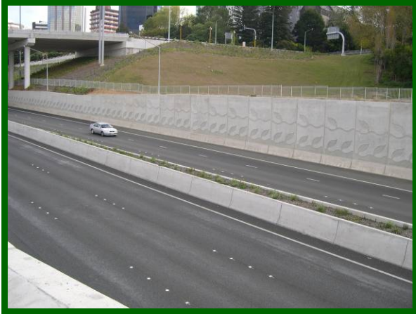
Figure 14: Patterns on retaining walls
