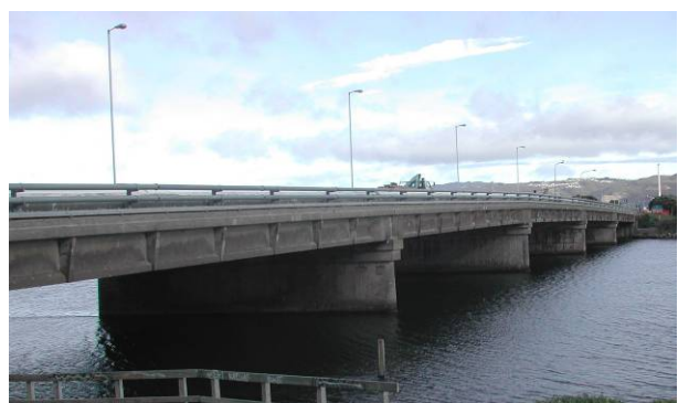
Figure 3: Hutt Estuary Bridge
