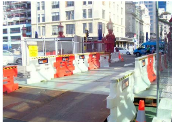
Figure 6 – Temporary ramp and structural support
