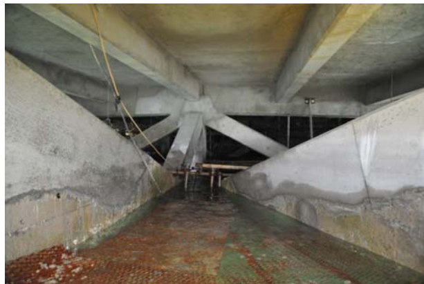
Figure 8 – Repairs using self compacting concrete.
