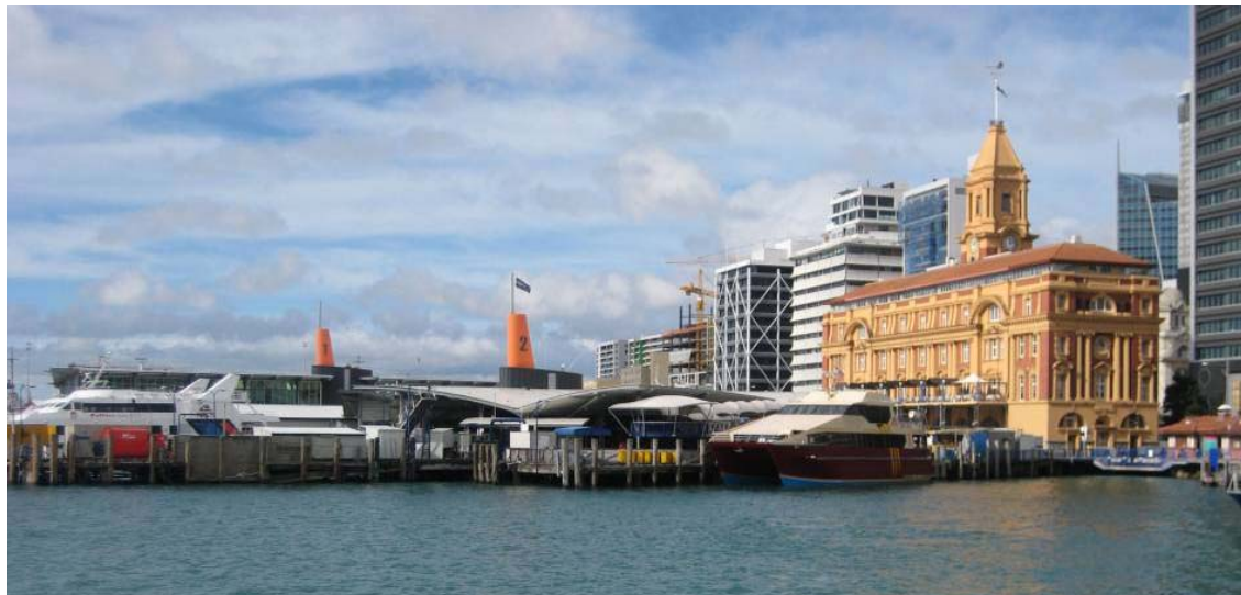
Figure 1 – Piers 1 and 2 of Auckland Downtown Ferry Terminal
