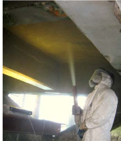
Figure 9 – Guniting of deck soffit.
