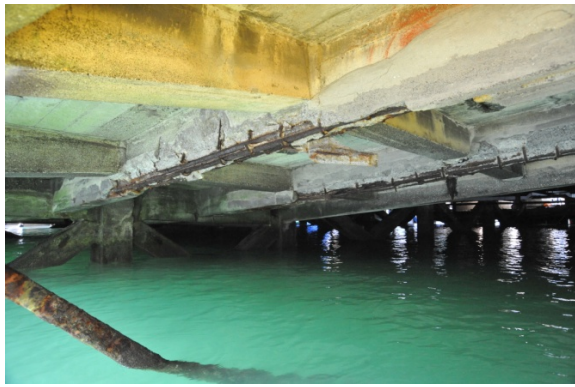
Figure 4 – Typical deterioration of beam, pile and cross brace elements requiring remedial work.
