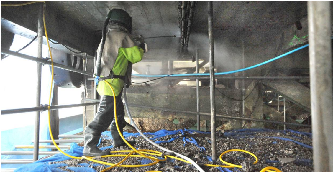
Figure 5 – Typical hydro-demolition of deteriorated concrete on a deck support beam.
