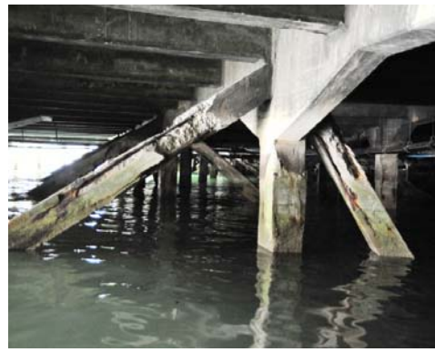
Figure 4 – Typical deterioration of beam, pile and cross brace elements requiring remedial work.
