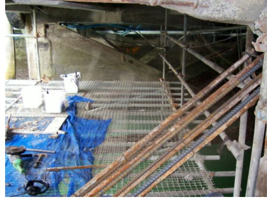
Figure 7 – Scaffold access platform
