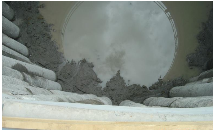
Exposed wall - pile with defects due to loss of workability prior to casing removal
