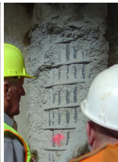
Exposed wall, membrane, dowels, , shotcrete lining wall and congested reinforcement
