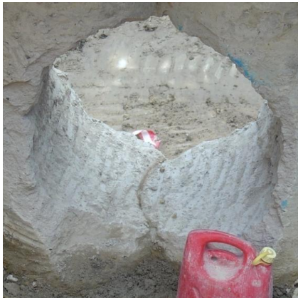
Exposed secant pile wall and pile interlock at pipe breakout location
