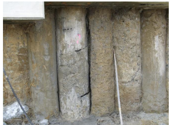
Exposed wall - pile with defects due to loss of workability prior to casing removal
