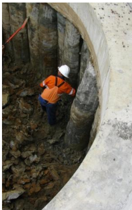
Misaligned secant piles, broken out piles and completed shaft prior to casting base slab
