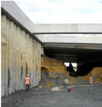
Polystyrene guidewall forms, installing casing and the exposed secant pile walls
