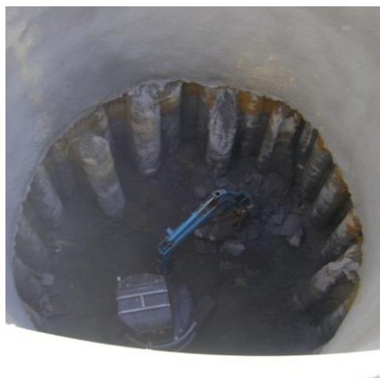
Misaligned secant piles, broken out piles and completed shaft prior to casting base slab
