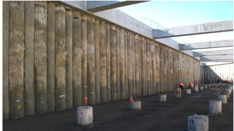
Polystyrene guidewall forms, installing casing and the exposed secant pile walls
