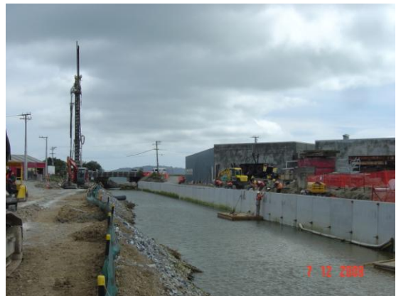
Arched soft piles / king piles exposed and with precast concrete facing panel
