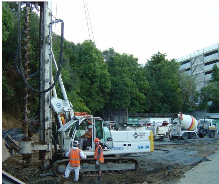
(Figure 4) CFA Piling
