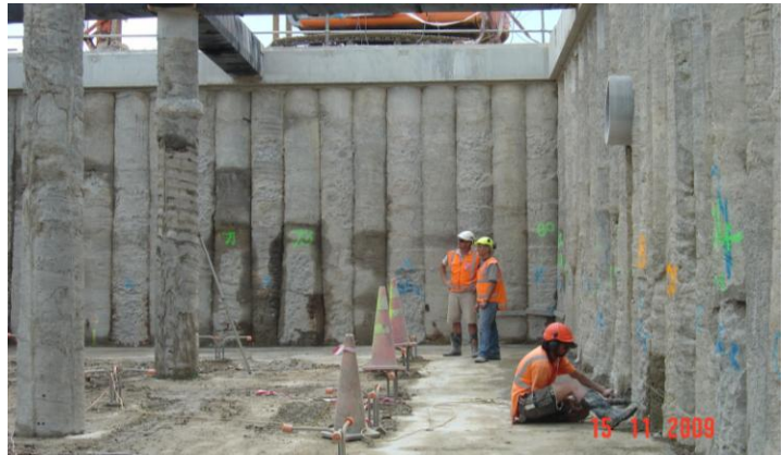
Exposed secant pile wall and pile interlock at pipe breakout location
