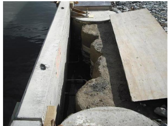
Exposed secant pile wall and pile interlock at pipe breakout location
