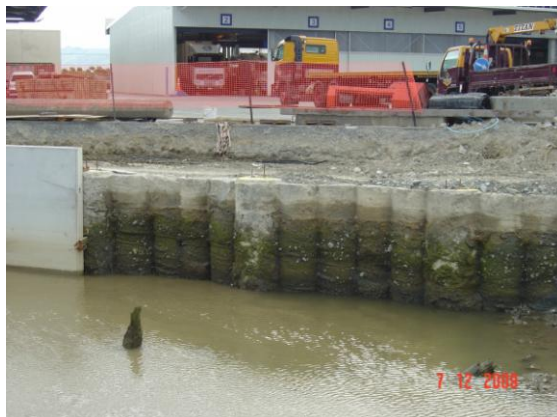
Arched soft piles / king piles exposed and with precast concrete facing panel
