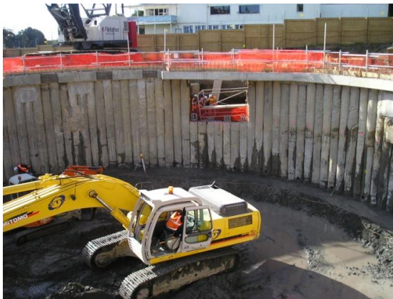
Exposed wall - pile with defects due to loss of workability prior to casing removal
