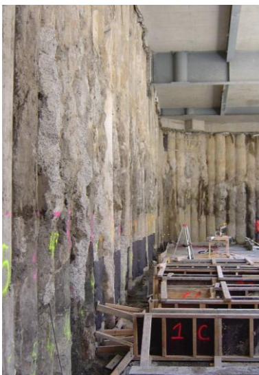
Exposed wall, membrane, dowels, , shotcrete lining wall and congested reinforcement
