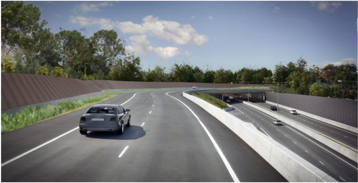
Fig. 2 View on Daylight Portal Western Connection
