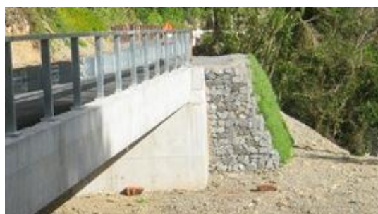
Figure 12: Green Terramesh Embankments
