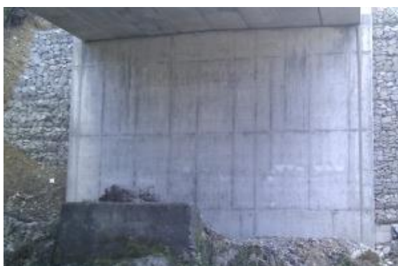
Figure 14: Bridge B 1/4 North Abutment
