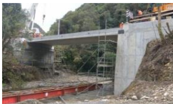
Figure 15: Bridge B 1/5 South Abutment
