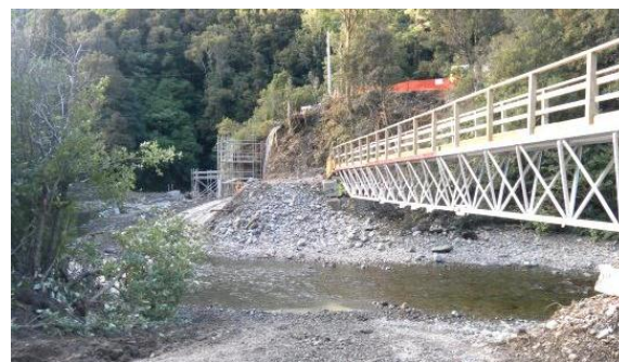
Figure 7: Temporary Pedestrian Bridges
