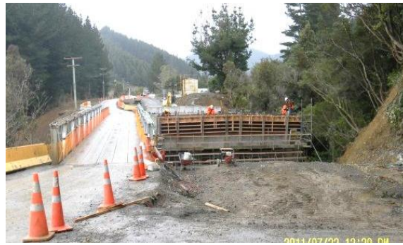
Figure 6: Bailey Bridge at B 1/4 Location
