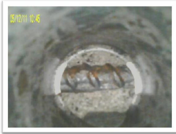
Figures 7 and 8. Borescope Images showing reinforcing bar encounters
