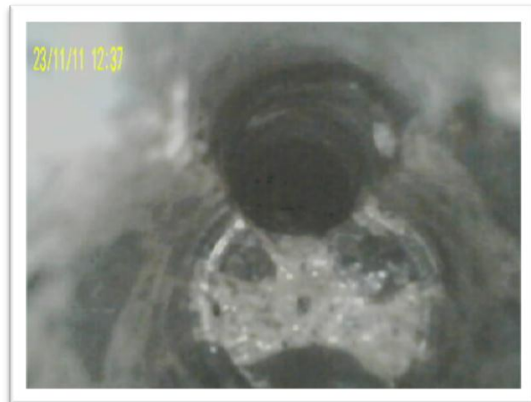
Figures 9 and 10. Pilot hole drilling at stressing strand duct locations
