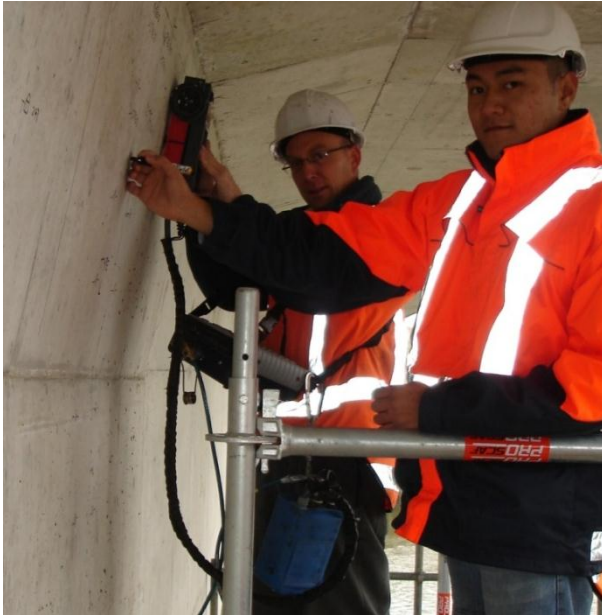
Figure 4. GPR scanning of structure
