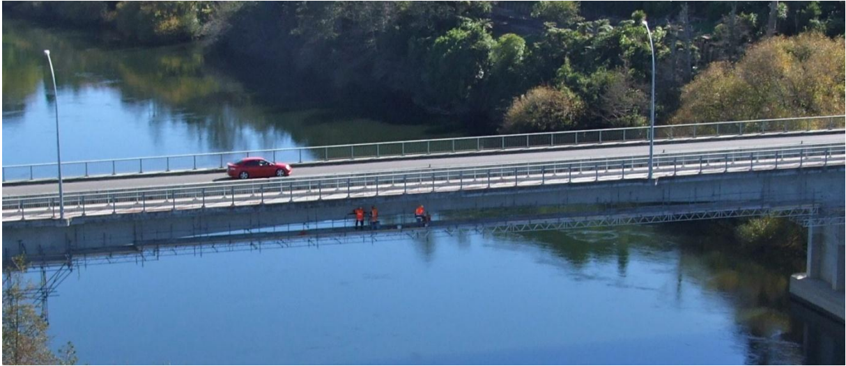
Figure 2. Main span suspended scaffold access
