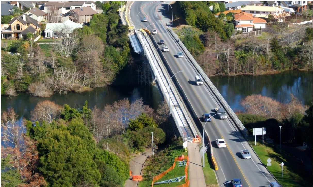
Figure 15. Aerial view of Pukete Bridge after stage one frame erection
