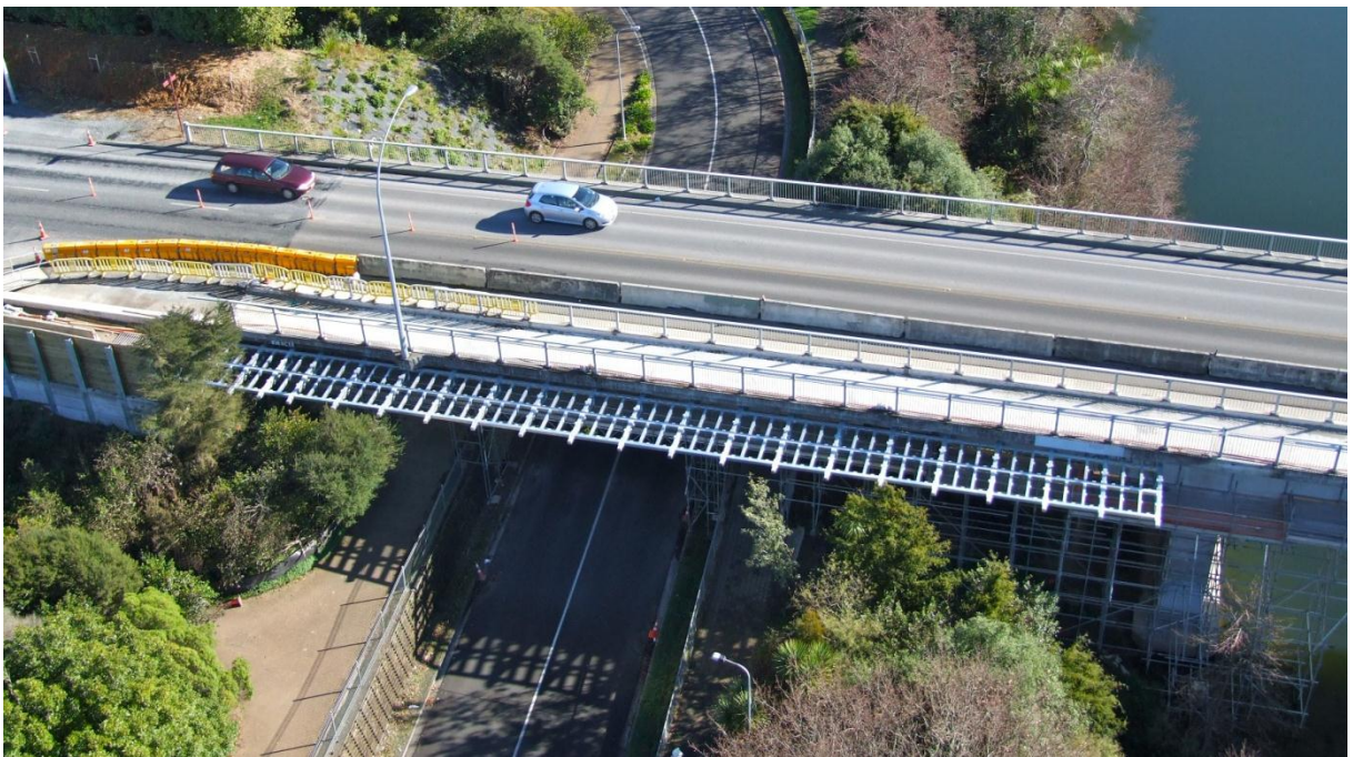
Figure 14. Stage One frames erected
