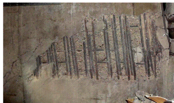
Spalled concrete in lap zone of stirrups - 2nd
