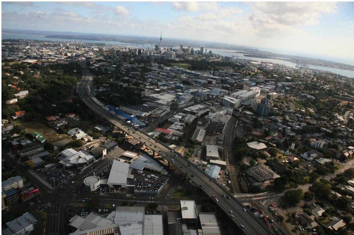
Figure 1. Aerial photograph showing the new southbound viaduct under construction.
