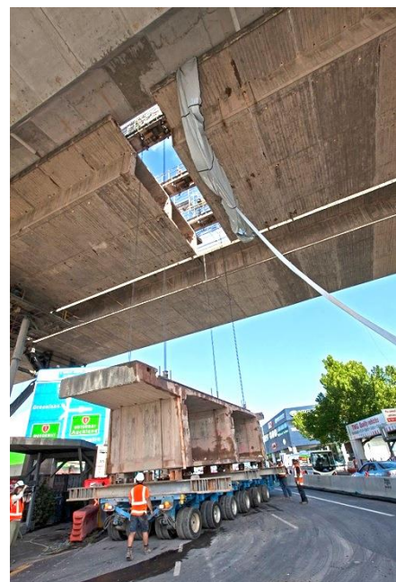
Figure 8 - Removal of closure segment over Broadway, Newmarket
