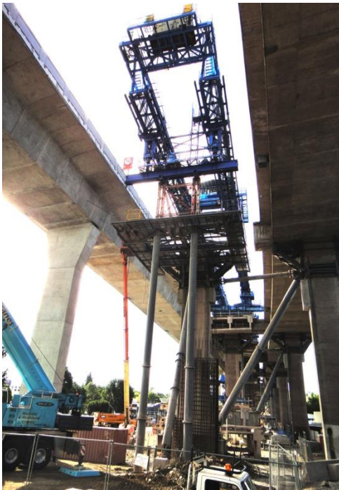
Figure 9. Deconstruction gantry supported on vertical props during pier segment removal.
