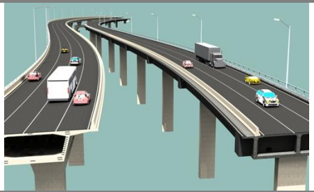
Stage 2 – Commission new southbound viaduct and deconstruct old southbound viaduct
