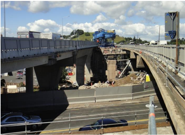
Figure 6. Deconstruction of the southbound viaduct.
