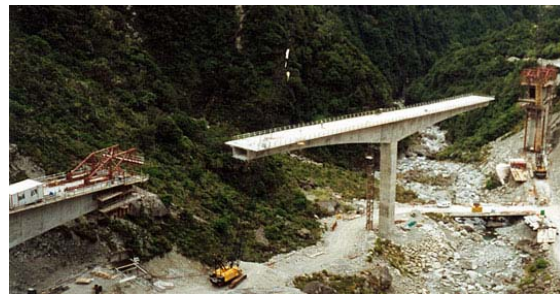
Figure 76. Otira Viaduct - Construction
