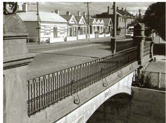
Figure 2. George Street Bridge
