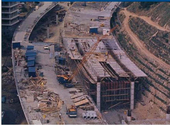
Figure 43. Shell Gully Bridge Construction
