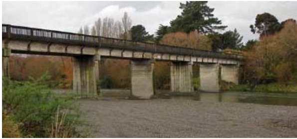
Figure 5. Waihenga Bridge, Martinborough
