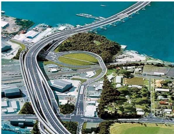
Figure 57. Chapel Street Viaduct
