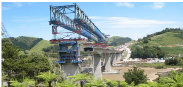
Figure 79. Waiwera Viaduct Construction
