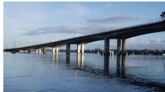
Figure 68. Upper Harbour Bridge Duplication
