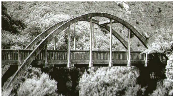
Figure 21. Tangahoe Valley Road Bridge
