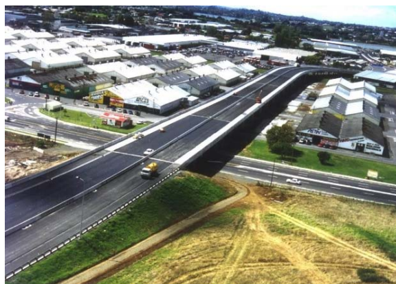
Figure 51. Sylvia Park Viaduct Aerial view
