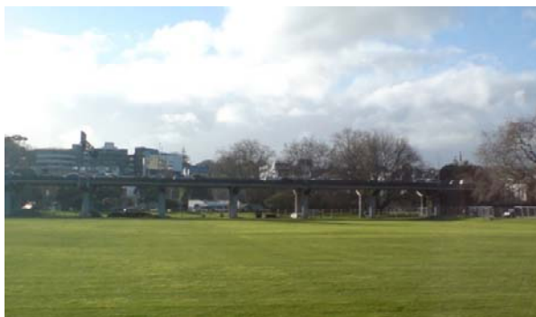
Figure 35. Victoria Park Viaduct
