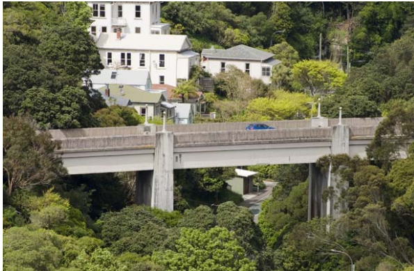
Figure 9. Kelburn Viaduct, Wellington
