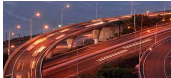
Figure 48. Night view of Ngauranga Flyover
