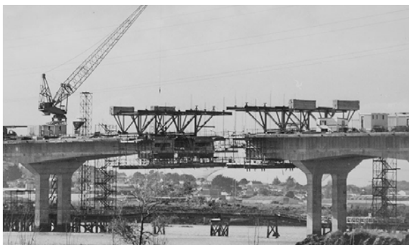
Figure 71. Mangere Bridge Construction 1980
