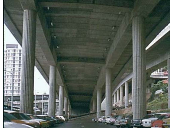
Figure 44. Shell Gully Bridge (underside)
