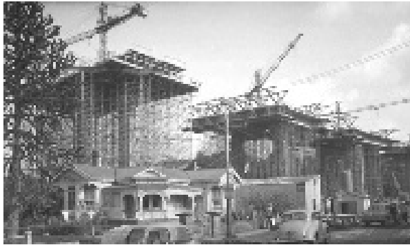
Figure 61. Newmarket Viaduct construction 1964
