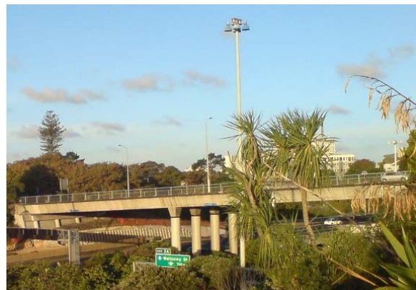
Figure 42. Symonds Street Bridge
