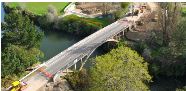
Figure 23. The Narrows Bridge
