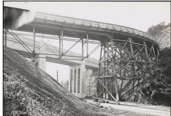
Figure 10. Old & New Kelburn Viaduct
