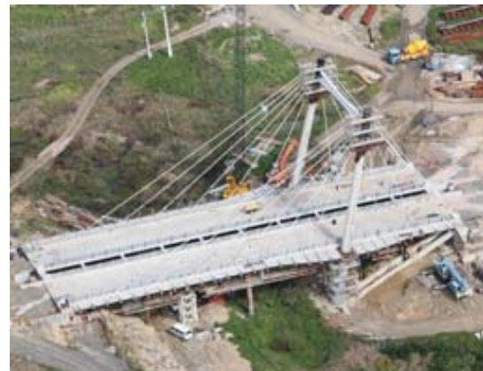
Figure 84. Ormiston Road Bridge Construction
