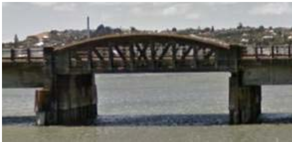
Figure 31. Westshore Bridge in Napier
