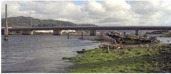
Figure 33. Hutt Estuary Bridge
