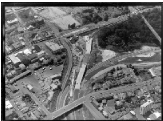
Figure 41. Symonds Street Bridge (1971)
