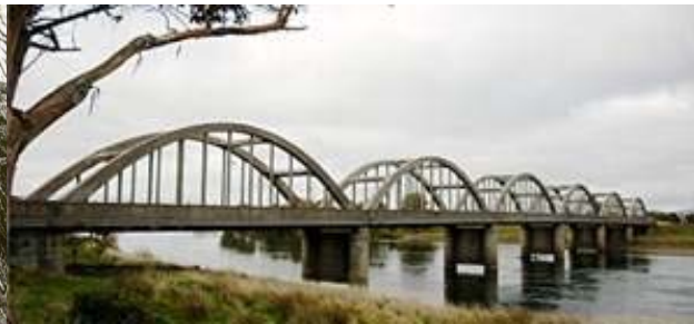
Figure 26. Balclutha Road Bridge (1935)
