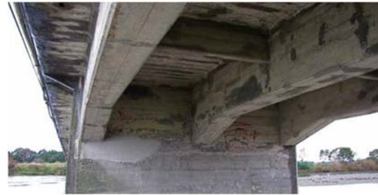
Figure 6. Waihenga Bridge, Pier beams connection
