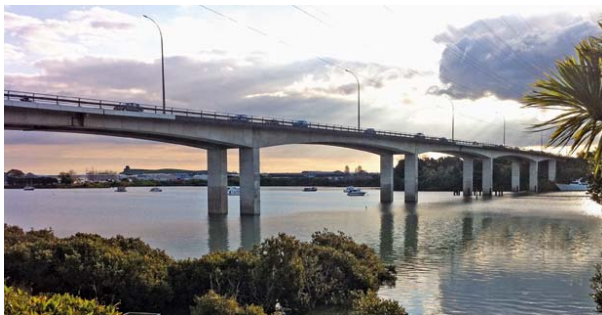
Figure 65. Waipuna Bridge (east View)
