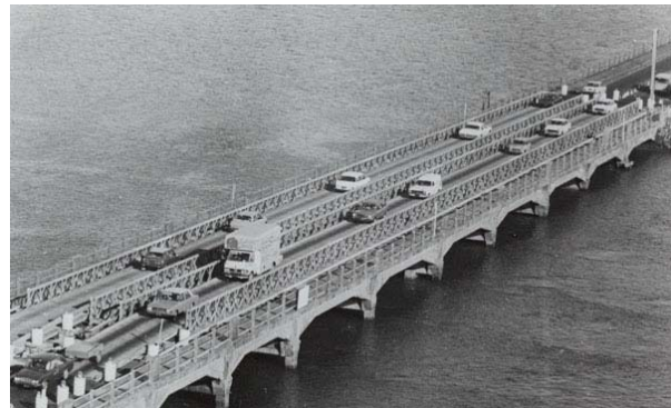
Figure 8. Old Mangere Bridge
