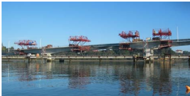
Figure 67. Upper Harbour Bridge Duplication Construction
