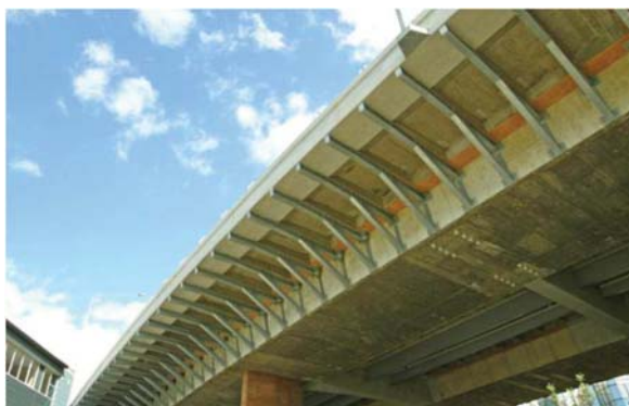
Figure 53. KPV-Cantilever deck strengthening with steel brackets
