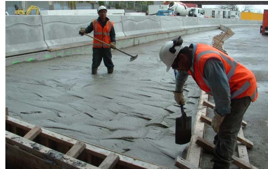
Figure 56. CMJ2-1 st Formcrete application
