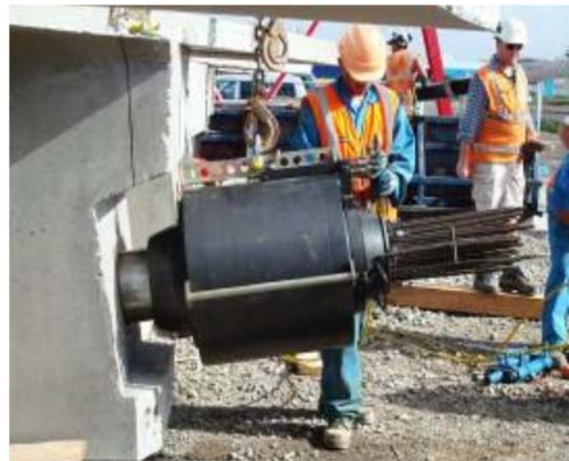
Figure 58. Post-tensioning Super T Beam
