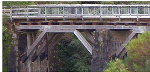
Figure 4. Ladle Bend Timber Bridge (1876)
