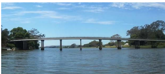
Figure 63. Clarence River Bridge
