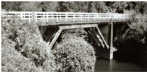
Figure 3. Tariki Road Concrete Bridge
