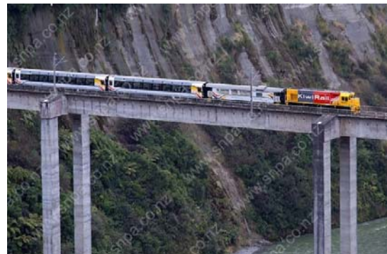
Figure 46. South Rangitikei Viaduct superstructure
