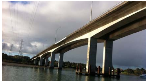
Figure 66. Waipuna Bridge (west view)
