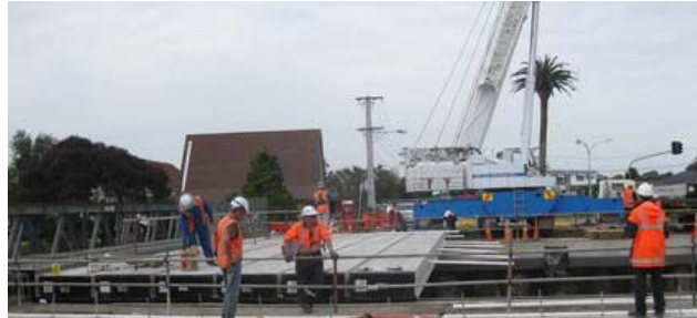
Figure 82. Papatoetoe Station Footbridge Construction
