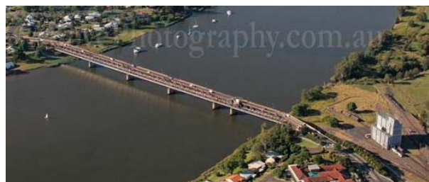
Figure 64. Clarence River Bridge
