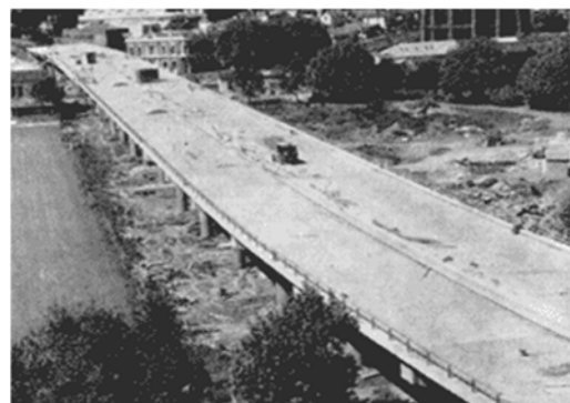
Figure 36. Victoria Park Viaduct Construction
