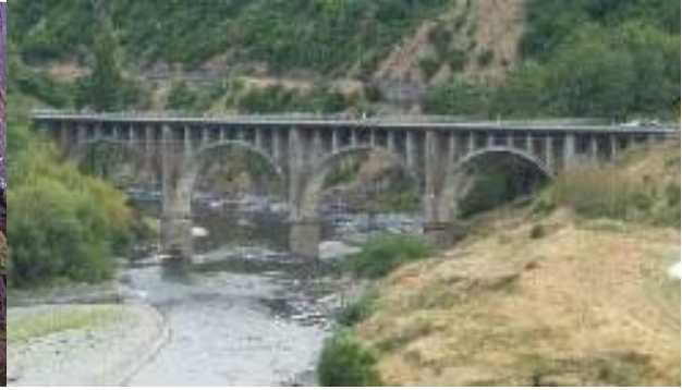
Figure 16. Manawatu Gorge Bridge
