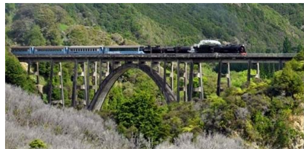
Figure 24. The Kopuawhara Railway Viaduct
