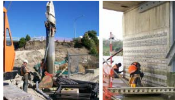
Figure 38. Cobham Bridge Strengthening
