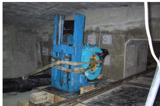
Figure 54. KPV- New external longitudinal post tensioning
