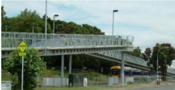
Figure 81. Papatoetoe Station Footbridge
