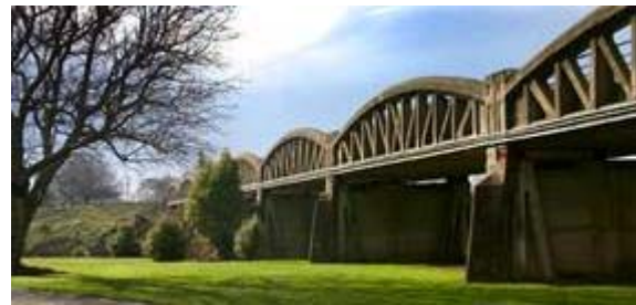
Figure 30. Opawa River Bridge
