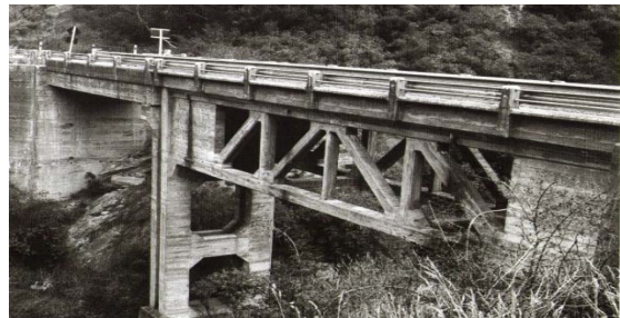
Figure 32. Gentle Annie Creek Bridge
