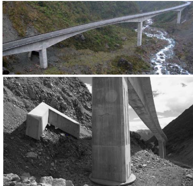
Figure 78. Otira Viaduct – Rockfall Protection
