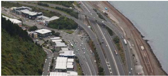
Figure 47. Ngauranga Flyover Bridge
