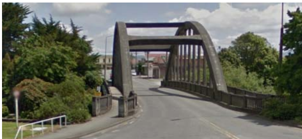
Figure 29. Mataura River Bridge
