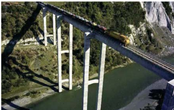
Figure 45. South Rangitikei Viaduct
