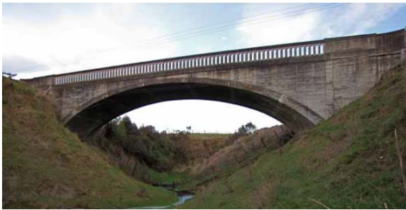
Figure 17. Parawhaiti Stream Bridge
