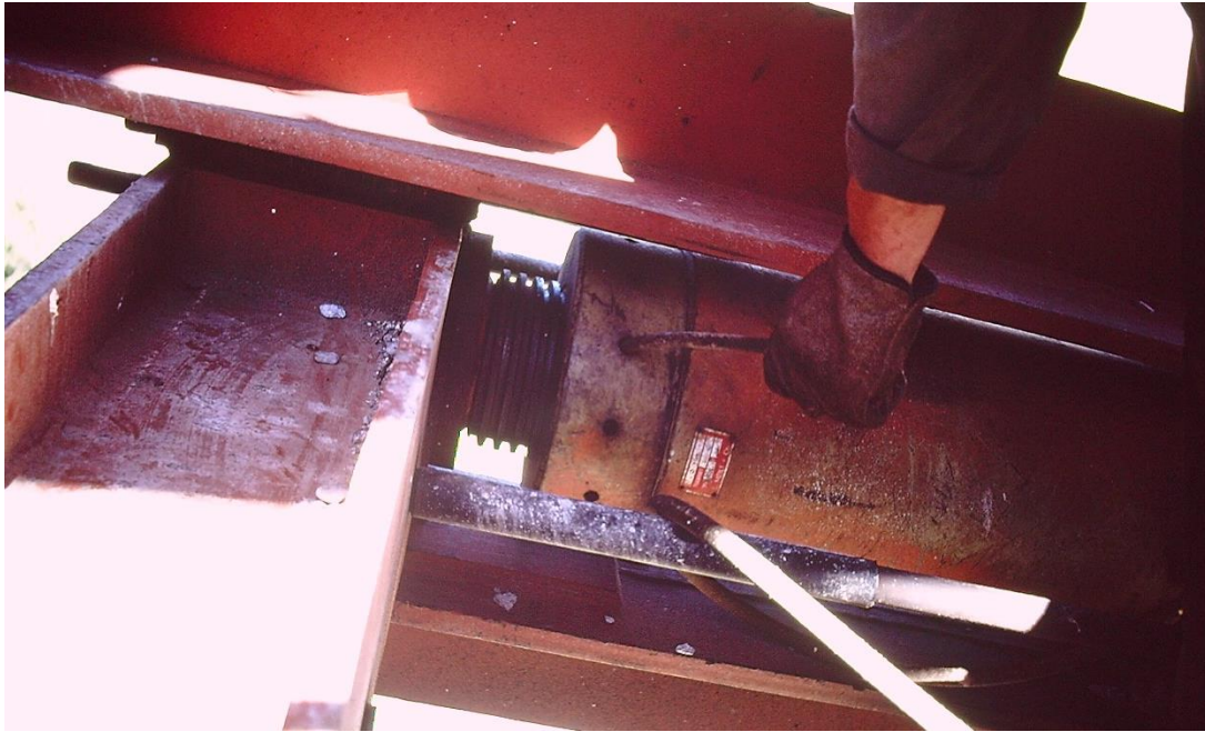
Figure 10 – Lock-ring jack for adjusting load in Macalloy bar understay system.
