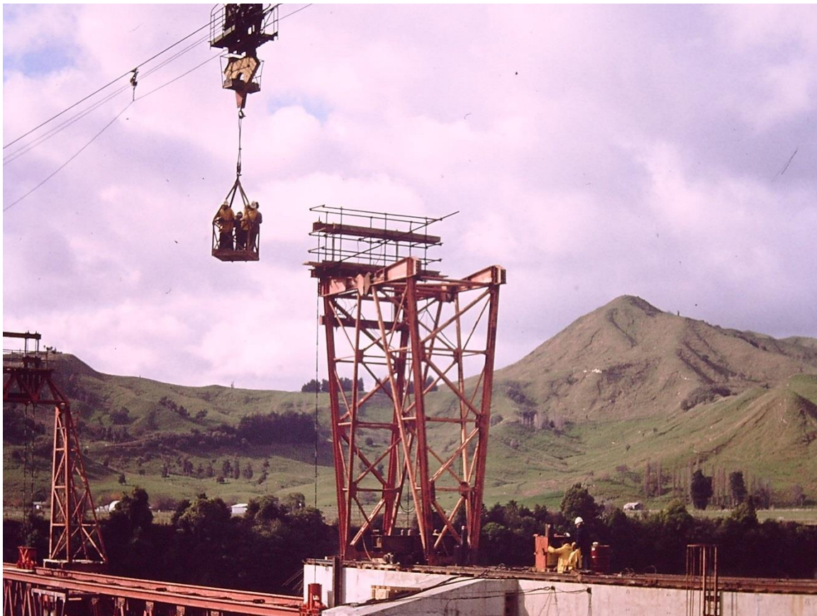
Figure 4 – the 3tonne capacity Blondin cable way was supported on towers spaced at 450m and delivered workers, equipment and concrete to any working level over a 14m plan width.
