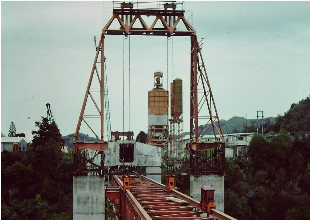
Figure 5 – Background from left to right: workshop, cableway tower slewed to left, 1m 3 CIFA batching plant, canteen, and office and control room for flying fox. Visible in the foreground are the temporary towers, transverse truss and hydraulic jacks at Pier 5 during assembly LG.
