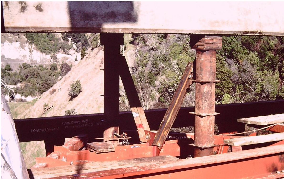
Figure 11 – Packing system and shims around hydraulic jacks supporting each segment until completed span post-tensioned.
