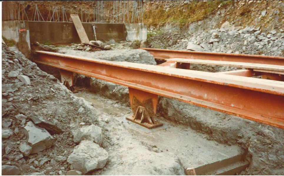
Figure 13 Sliding bearings under top chord nodes near North Abutment
