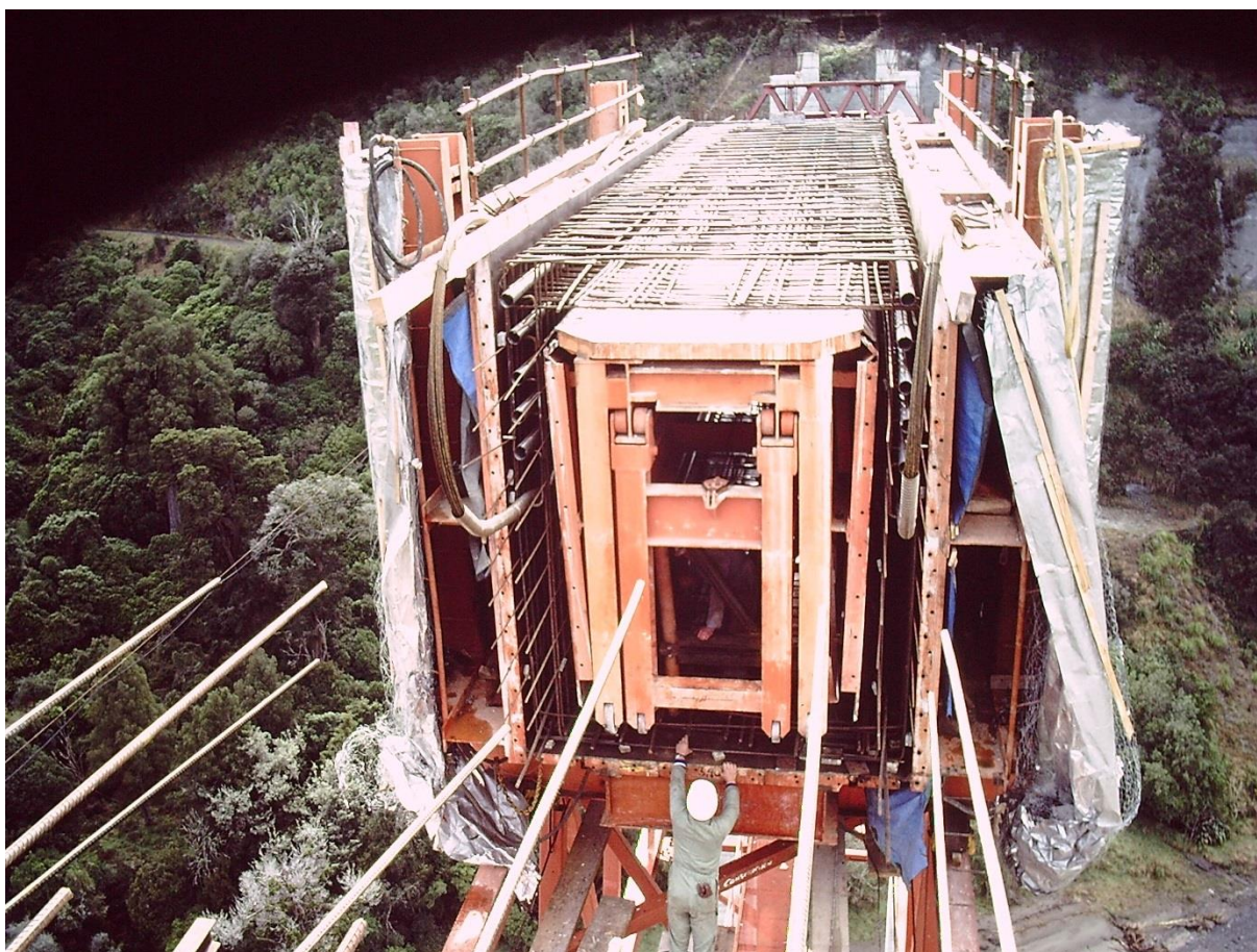
Figure 9 – 80tonne steel form – temporarily over-advanced, cleaned, oiled and rebar installed for cantilever segment while waiting for piercap formwork and rebar to installed concurrently. Rolled back to join piercap form prior to combined pour.
