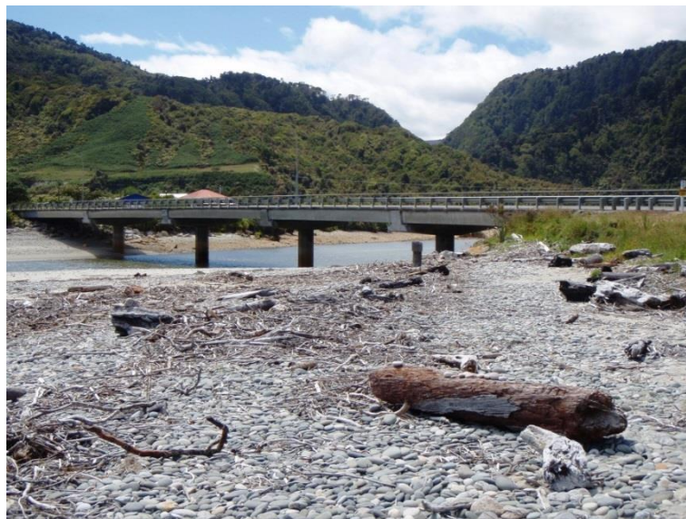
Figure 2. General view of the Ngakawau River Bridge & environs, seen from the Westport (south) side of the bridge.
