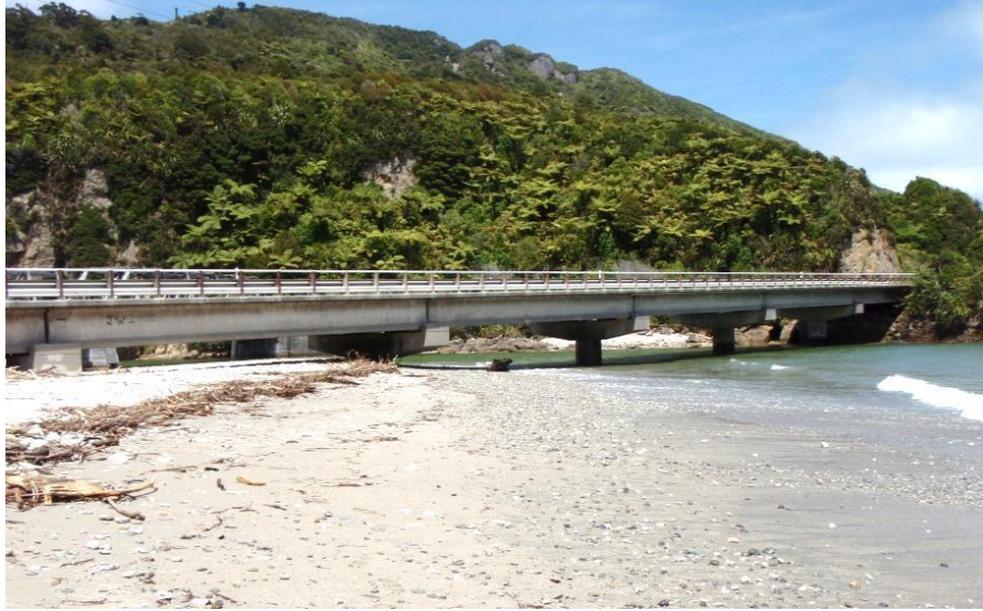
Figure 1. General view of the Fox River Bridge & environs, looking southward in the direction of increasing R.P.
