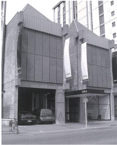
Figure 7: The Canterbury Society of Arts building is a commanding presence in Gloucester Street with beautifully daylighted exhibition spaces
