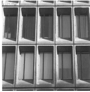
Figure 11: Detail of the precast concrete cladding panels on the SIMU building
