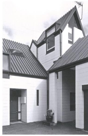
Figure 6: Peter Beaven was influenced by European hill towns and medieval laneways with the planning of Tonbridge Mews.
