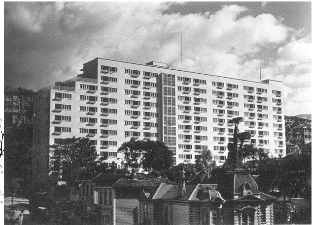
Figure 2: The design of the Dixon Street Flats was linked closely to Austrian architect Ernst Plischke
