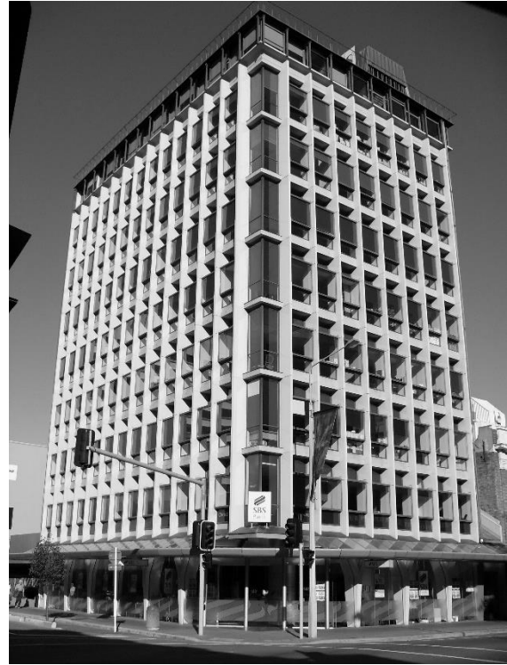
Figure 12: Manchester Unity, certainly one of Peter Beaven's finest buildings in the city. Prior to the earthquakes the building had undergone extensive renovation.
