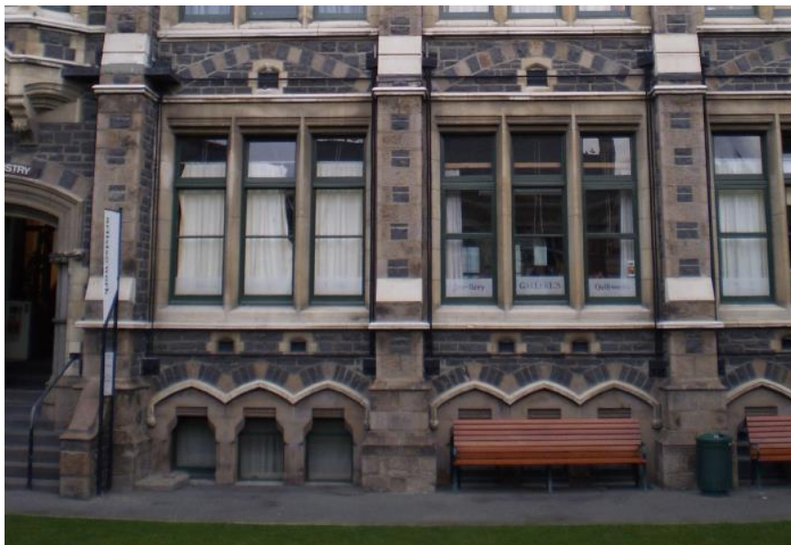
Figure 3. Photograph Showing Post Tensioning to the Chemistry Building
