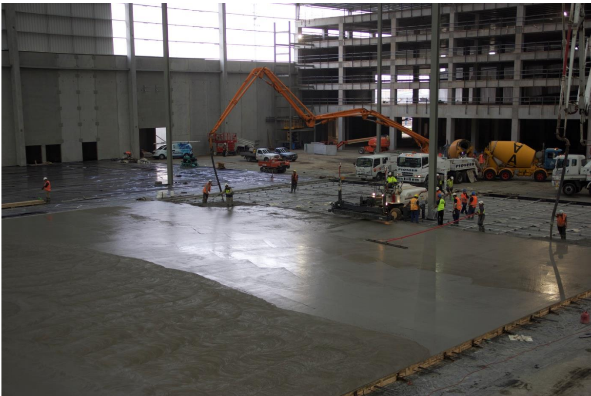
Figure 6 Large bay post-tensioned floor pour at JPL
