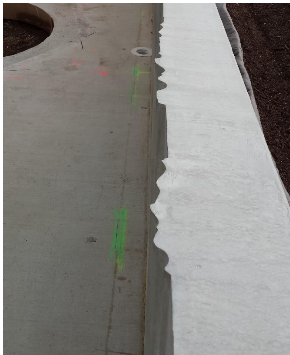
Figure 6 Example of relief generated by timber profile
