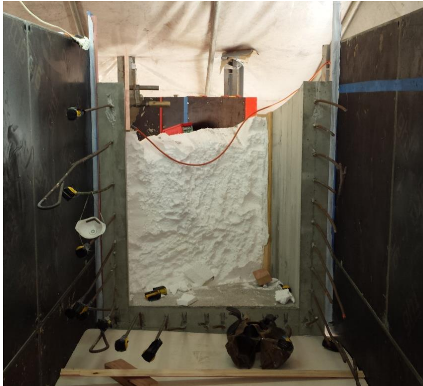
Figure 8 – showing polystyrene core, timber form, pour staircase and protruding reinforcing for bridge
