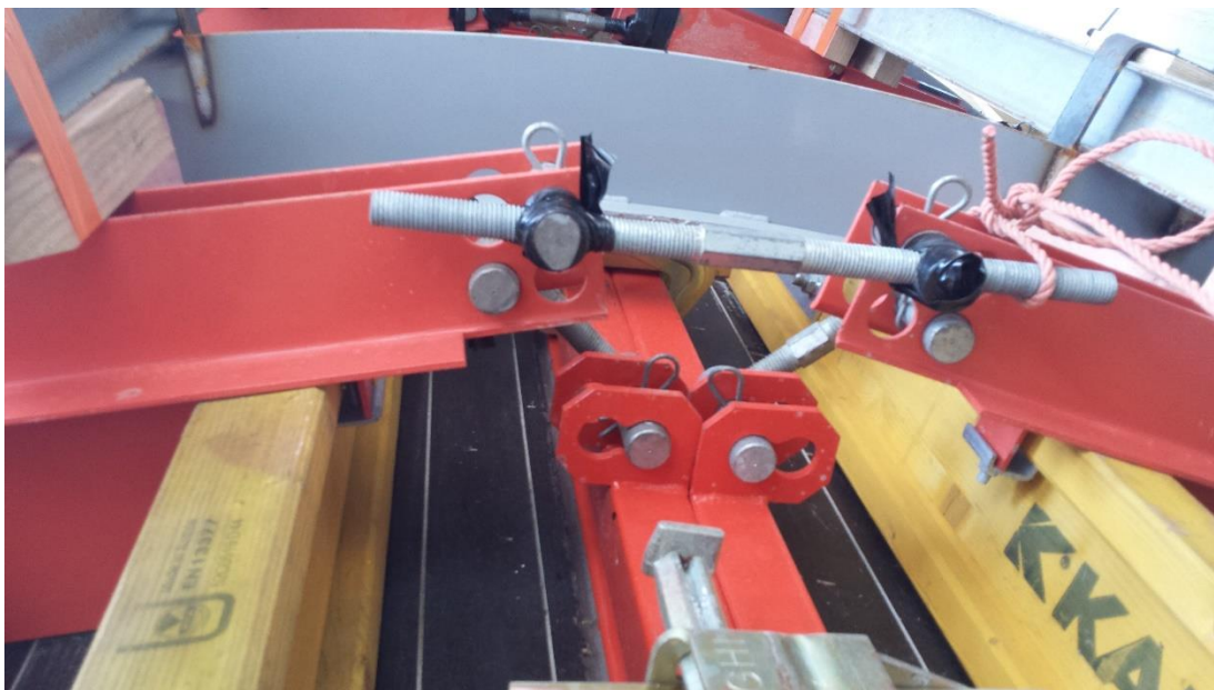
Figure 9 Formwork set up on external barrel
