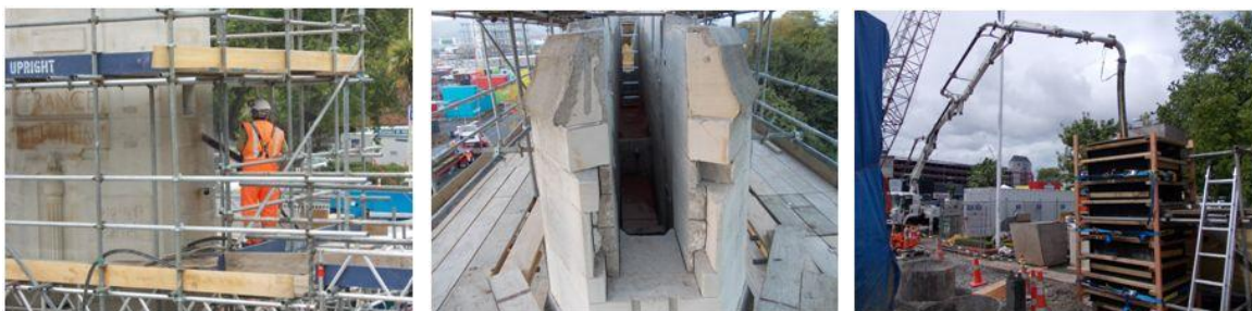
Figure 8. (L-R) Stonemason working, Limited space inside Major Arch, Concrete Test Pour
