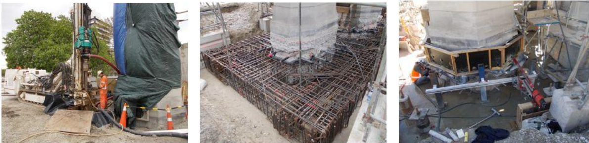
Figure 6. (L-R) Piling Work, Pile Cap reinforcement, Rocking Collar Coring
