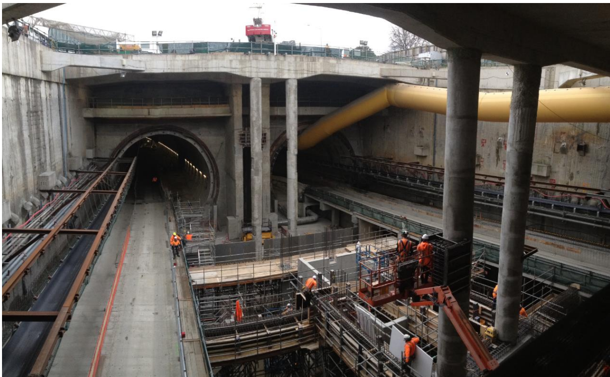
Figure10. Construction of the internal structure through the turnaround zone
