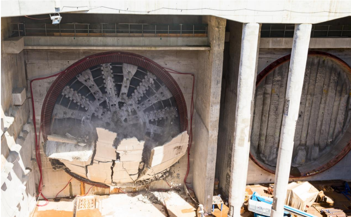
Figure 9. TBM breakthrough
