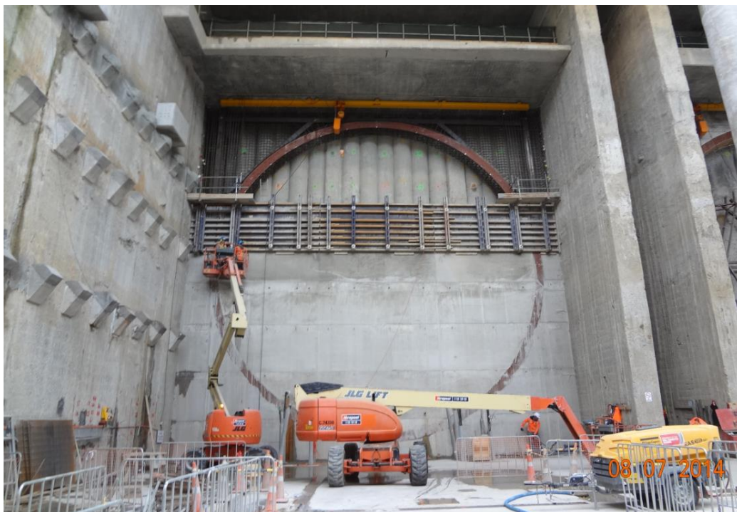
Figure 8. Facing Wall Construction
