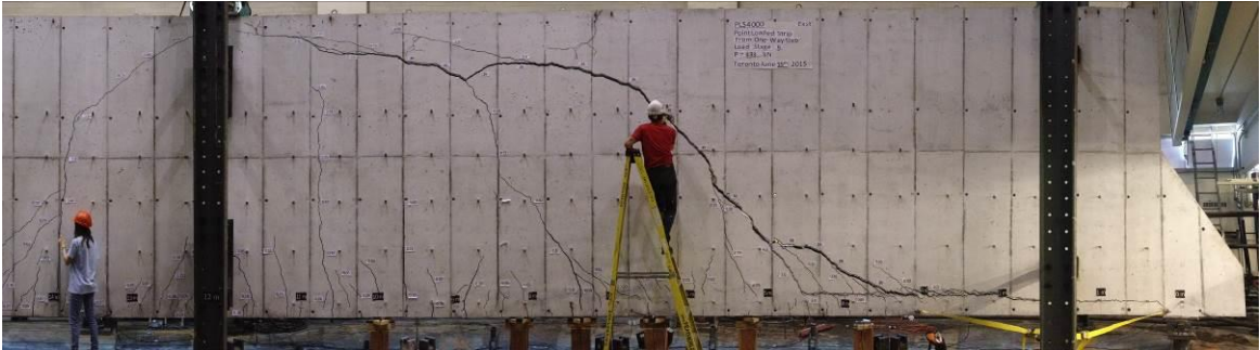
Figure 8. East span of PLS4000 after failure
