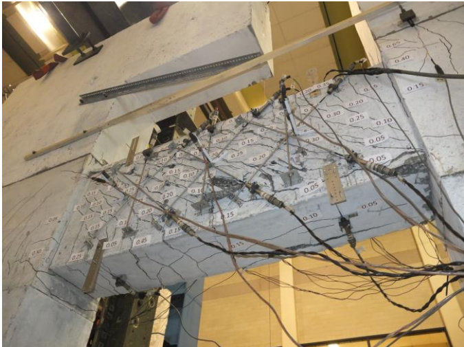
Figure 16. Instrumentation on back face, wall-to-wall displacement rod.
