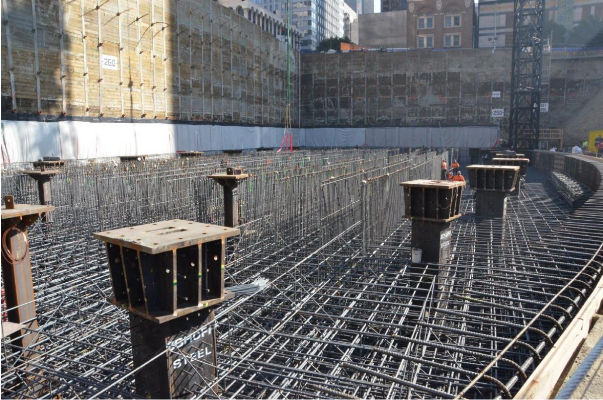
Figure 1. Reinforcement in mat foundation of Wilshire Grand
