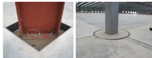
Figure 4. Typical isolation joint
