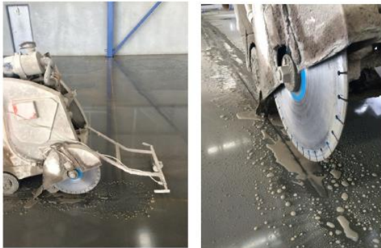
Figure 23. Saw-cutting process
