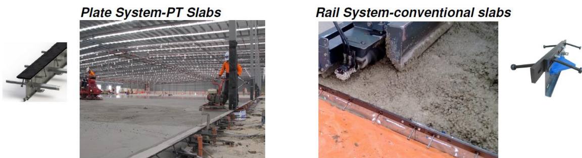
Figure 20. Edge protection – plate system Vs. rail system
