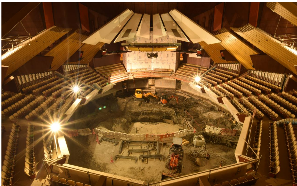
Figure 9: Inside view of Auditorium in preparation for the new raft slab foundation (photo dated May, 2016).
