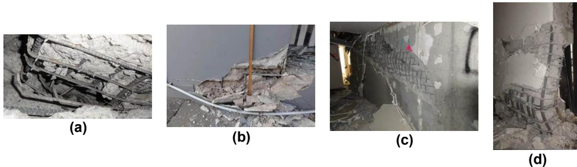
Figure 1: Observed Failure modes of structural walls during past earthquakes: (a) Bar yielding followed by bar rupture (b) Toe crushing (c) Diagonal shear (d) Compression failure and buckling (Kam et al., 2011)
