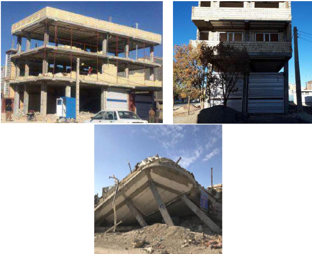
Figure 6. Torsion Failure
