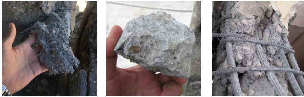
Figure 7. concrete without sand, grains or discrete aggregate
