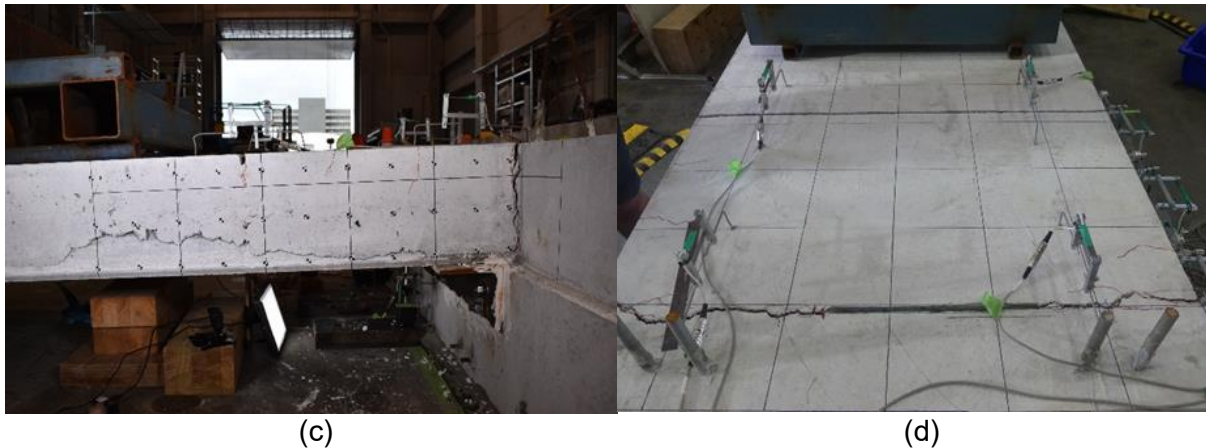
Figure 8: Specimen 3 at -3.5% Drift (c) and Specimen 3 Topping With Saw-Cut (d)
